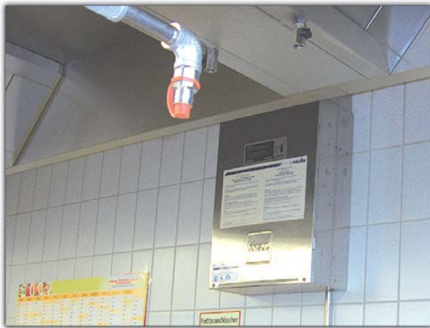
External fire-extinguishing system as wall-mounted unit
