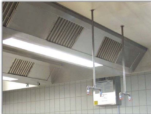
Fire-extinguishing system integrated into the ventilating ceiling
